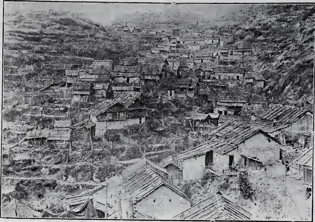
A typical aborigine village, perched high up on the mountain side. The low one-story houses are made of sun-dried brick, and roofed with bark or tiles. Their floors are made of earth, and as there is almost no furniture, serve the purposes of chairs, tables, beds and storage places for belongings. In many of them cooking is done in a hole in the floor, in a pot supported by stones. The water used in some villages is carried from springs half a mile down the mountain side, or taken from stagnant pools accessible to live stock. From these villages the people go daily to their fields, some of which are two or three miles away down the mountain sides, and climb back again in the evenings. From the villages, farm products and fuel must be carried a minimum of seven miles to market, and if not sold, carried back.
